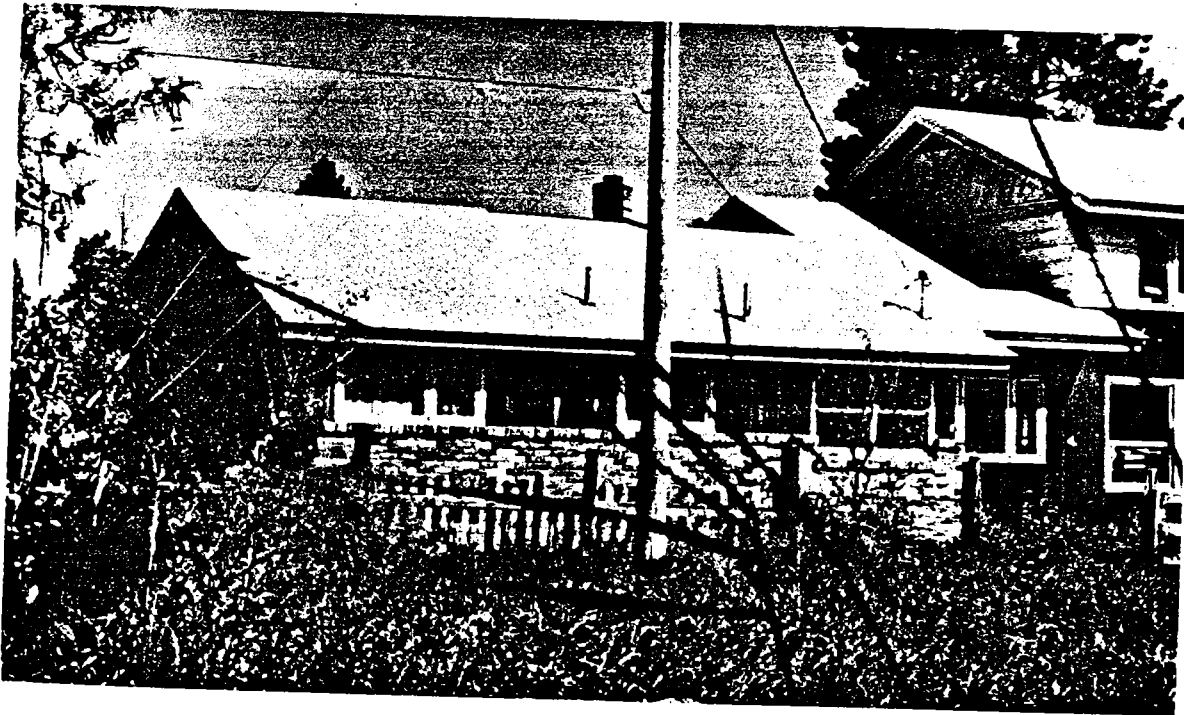
Figure 28.—Test structure 61, near a coal mine.
