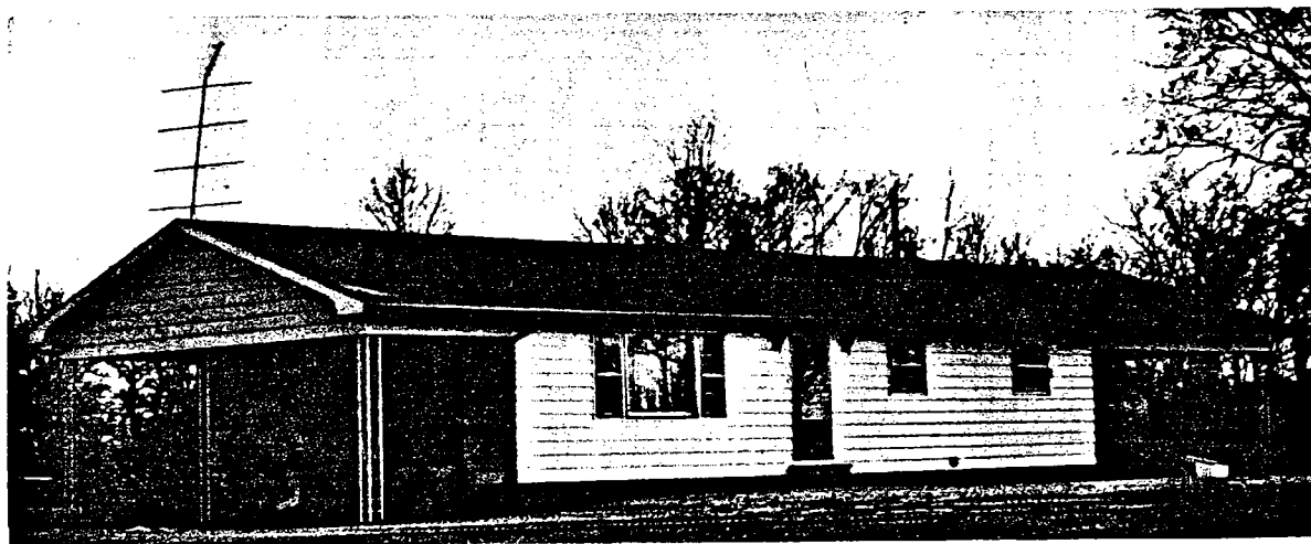
Figure 17.—Test structure 21, near a coal mine.
